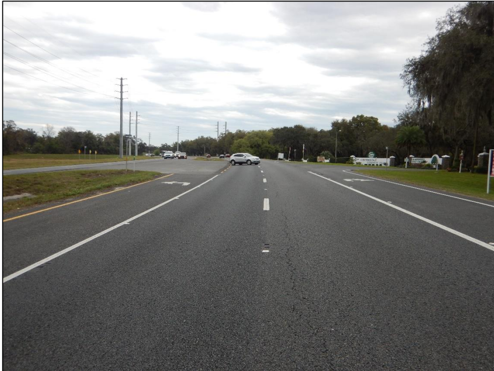
Exhibit 3: Looking east into the intersection along SR 44
