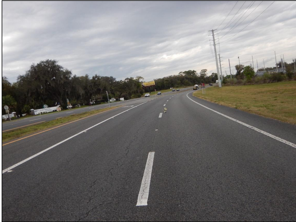
Exhibit 1: Looking west into the intersection along SR 44
